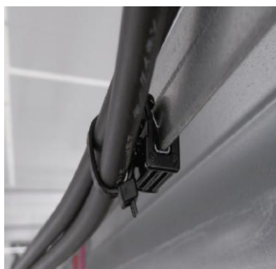
Example of utilizing wire clips and cable ties to manage wires along module frames
